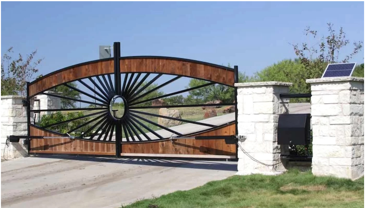
Proper Solar Panel Installation Paired with an Automatic Swing Gate Opener
